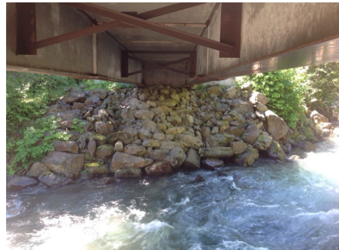
Right Bank Abutment when facing downstream
