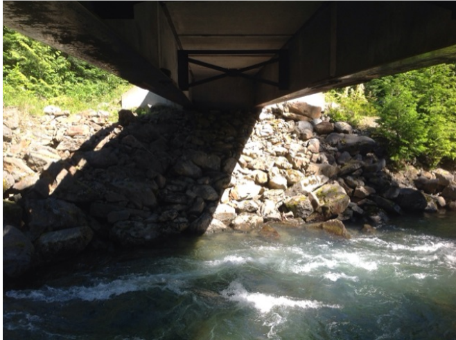
Left Bank Abutment when facing downstream
